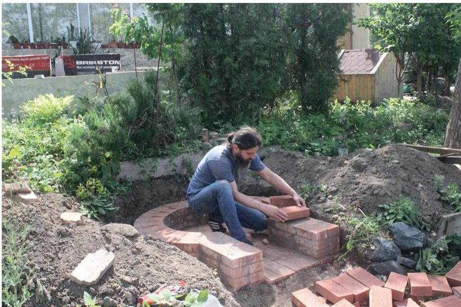
Fig. 2. *Work steps for the construction of the oven.*
