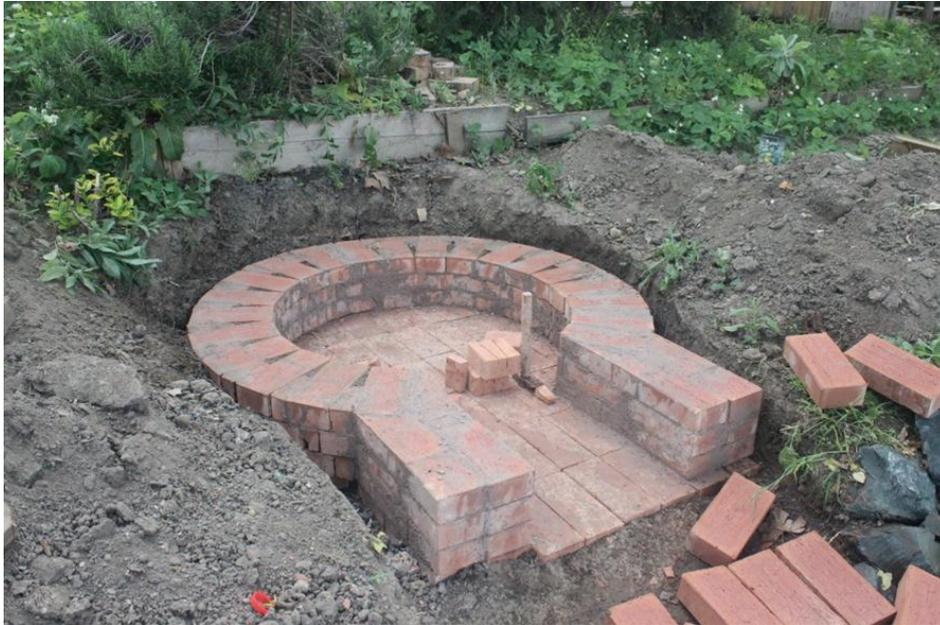
Fig. 1. *Construction of an archaic bicameral brick oven*
